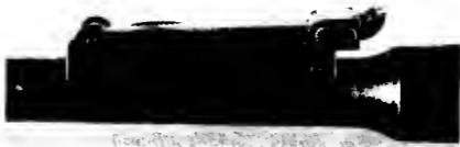
FIGURE 16. REAR SIGHT FOR RIFLE M1891/30 (SIDE VIEW).
